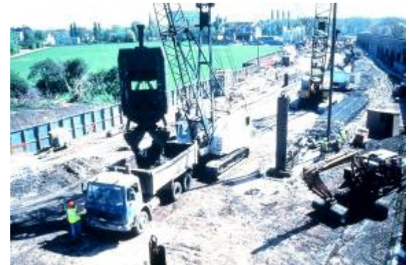
Building the DLR
