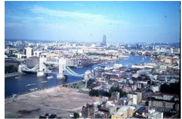
Docklands – looking east
